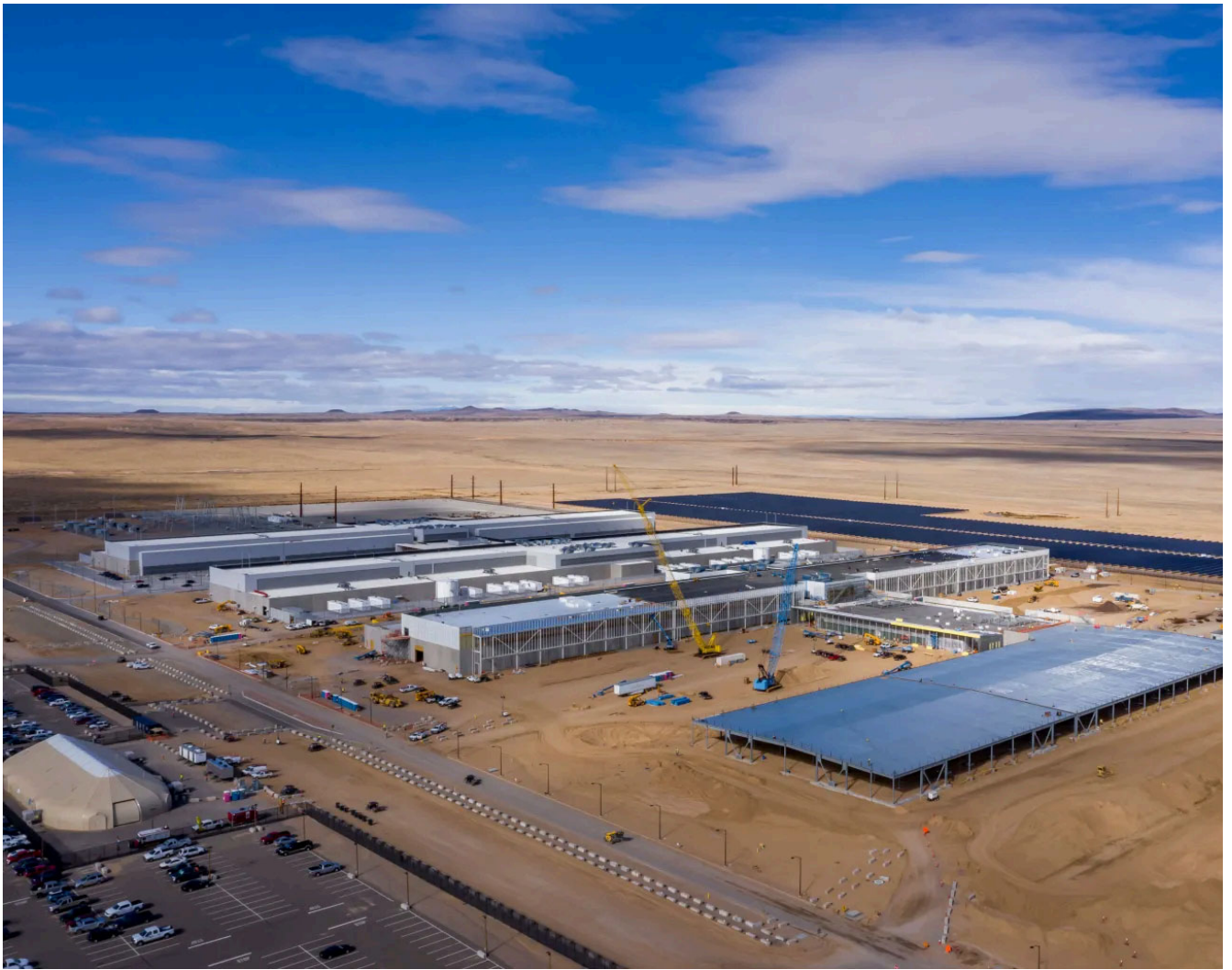
Our newest data center in New Mexico.
