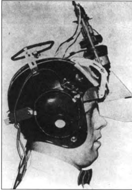
Figure 2.9 The Philco Headsight from 1961. (From Comeau and Brian [1961] )
