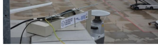
Figure 7. LiDAR sensor mounted at Dresden airport
