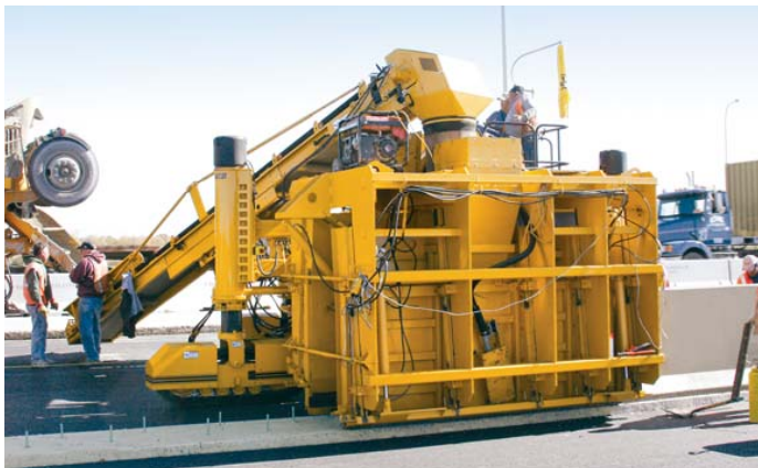
P.T. Ferro's barrier mold is built with double variable capabilities so each side of the wall can be adjusted for height.
