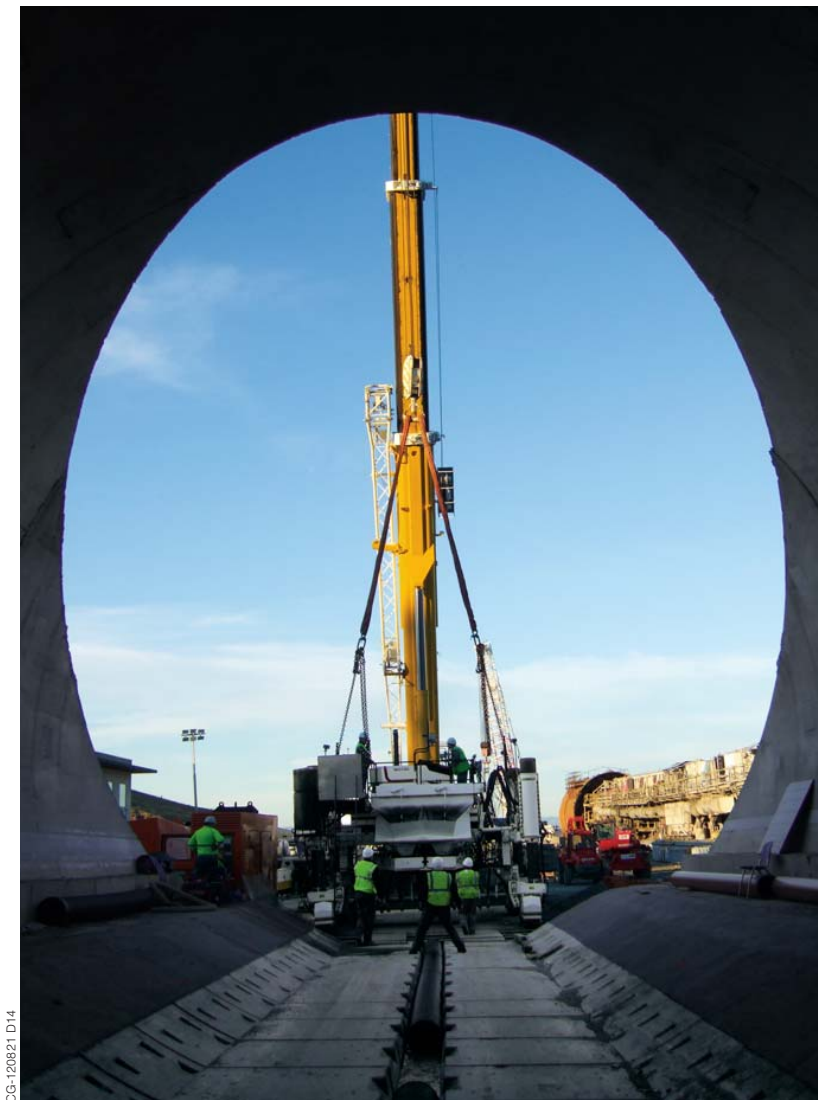
The Commander III four-track was lifted by crane into the tunnel at the beginning of each of the two tunnels.
