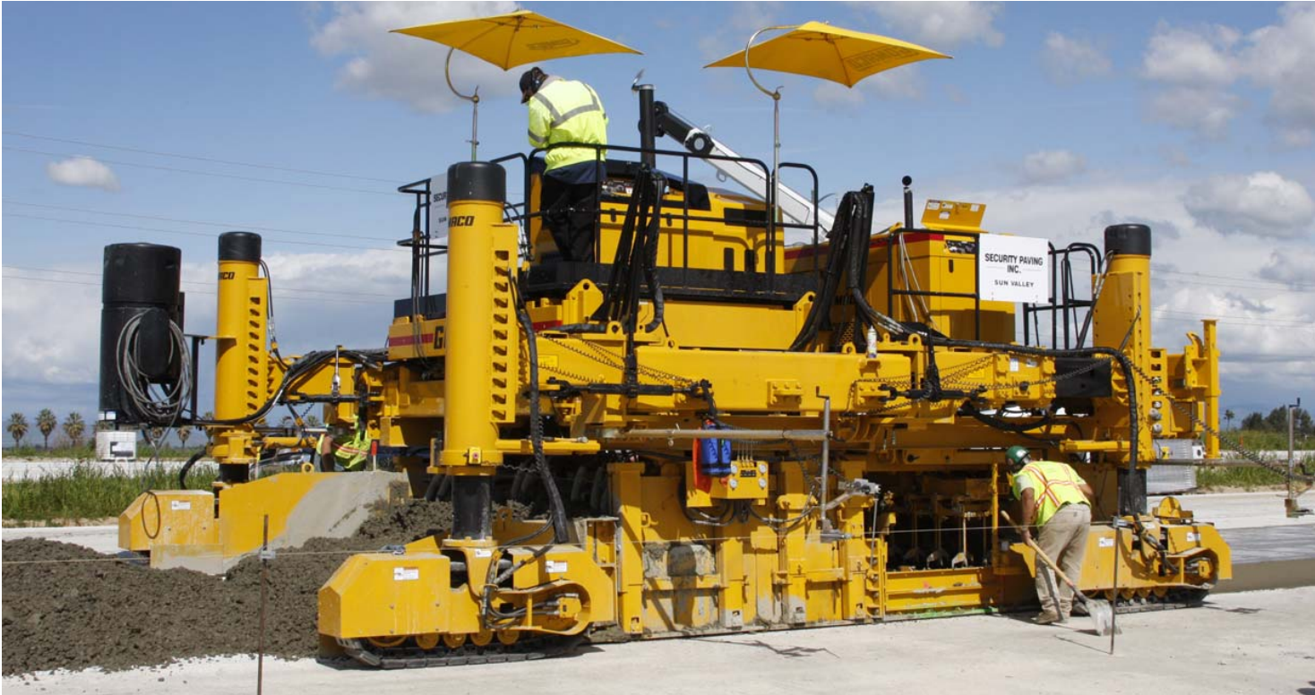
The Commander III four-track with IDBI attachment slipforms a new lane for a roadway project in Fresno, California.
