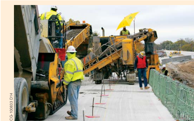
The first step to the sound wall is slipforming a moment slab. The slab features extra steel reinforcing slipformed into the concrete. The steel caging for the barrier wall is anchored to the steel in the slab. Extra supports for the sound wall are incorporated into the wall's steel cage. The posts that support and hold the sound wall panels are then bolted to the supports after the concrete wall has cured.
