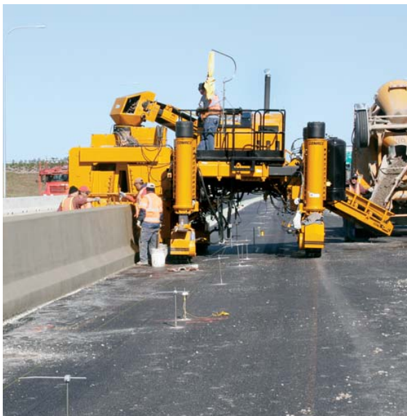
Stringline is set underneath the Commander III and out of the way of the finishers.
