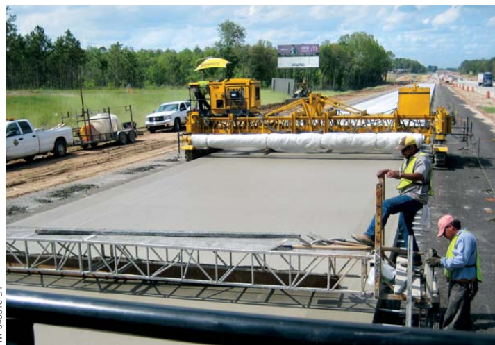
A T/C-600 texture/cure applied a tine finish and white spray cure.
