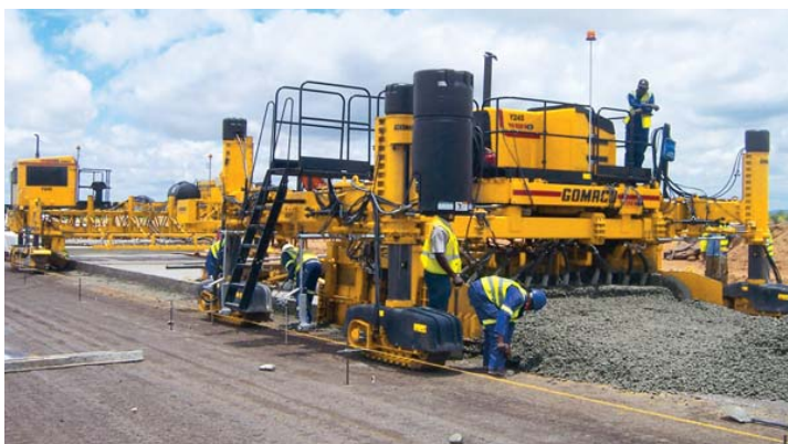
WBHO slipforms a new runway at the Sir Seretse Khama International Airport near Gaborone, Botswana. They are using a new Commander III four-track paver and a T/C-600 texture/cure machine to pave the five meter (16.4 ft) wide passes.
