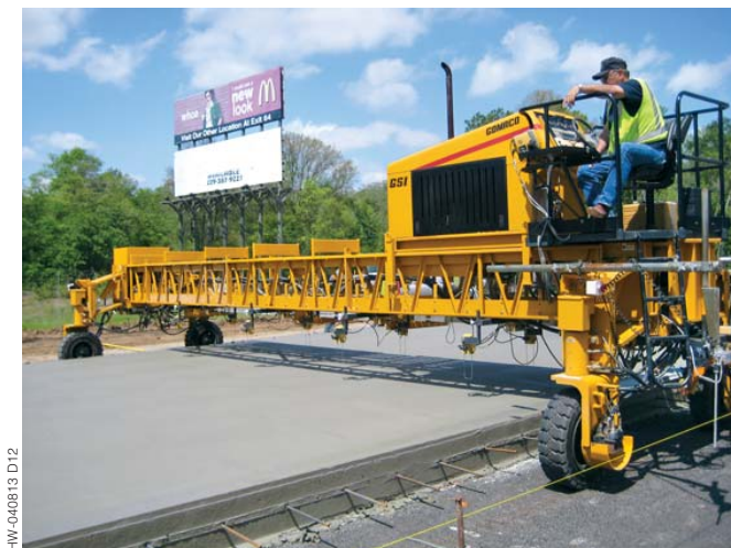
A GSI followed the paver providing instant rideability readings.
