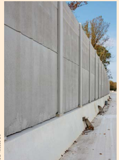
The first step to the sound wall is slipforming a moment slab. The slab features extra steel reinforcing slipformed into the concrete. The steel caging for the barrier wall is anchored to the steel in the slab. Extra supports for the sound wall are incorporated into the wall's steel cage. The posts that support and hold the sound wall panels are then bolted to the supports after the concrete wall has cured.
