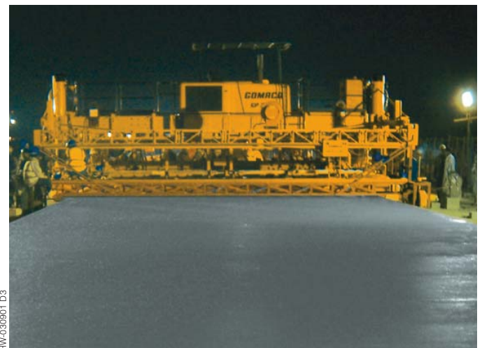
Orascom Construction Industries paves at night a new apron with their GP-2600 two-track paver at the Borg El Arab International Airport in Alexandria, Egypt.
