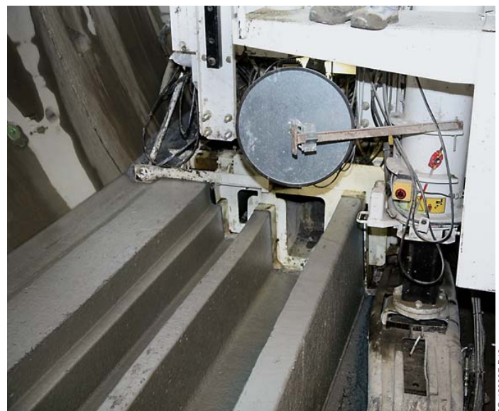
The double 'U' channel was designed to hold water pipes for fire protection and also house electrical cables.
