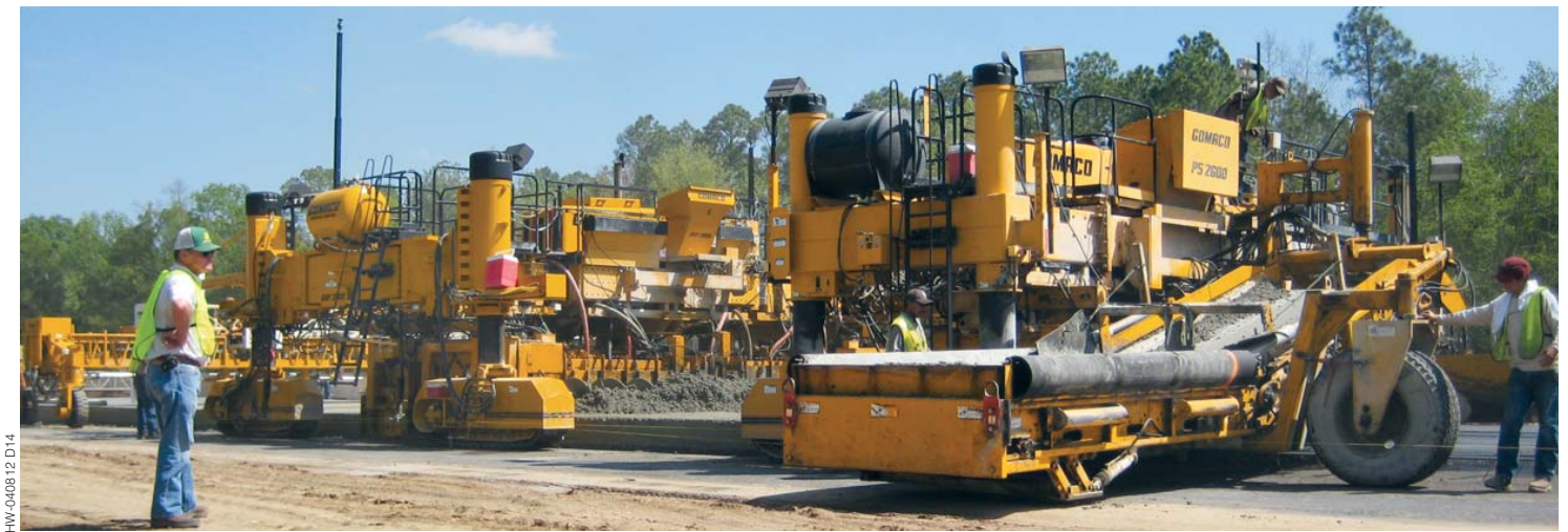
Scruggs PS-2600 placer/spreader and GHP-2800 paver are guided by the Leica stringless system. The GSI and T/C ran on stringline.
