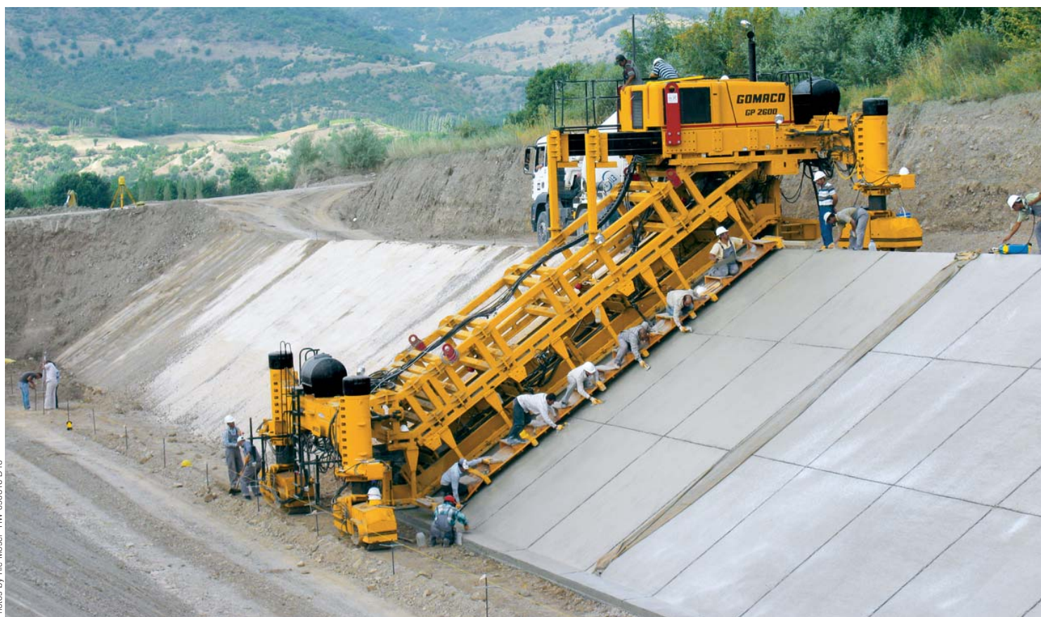
The GP-2600 with a front-mounted chain trimmer slipformed a new canal between Amasya and Tasova in northern Turkey.
