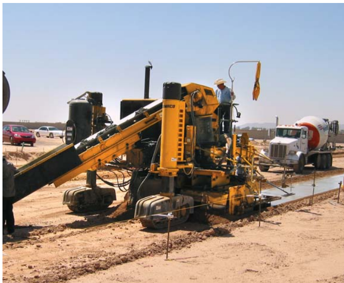
A total of 160,000 linear feet (48,768 m) of curb and gutter and monolithic sidewalk and curb and gutter was slipformed on the project. All of the concrete was done with Commander IIIs.
