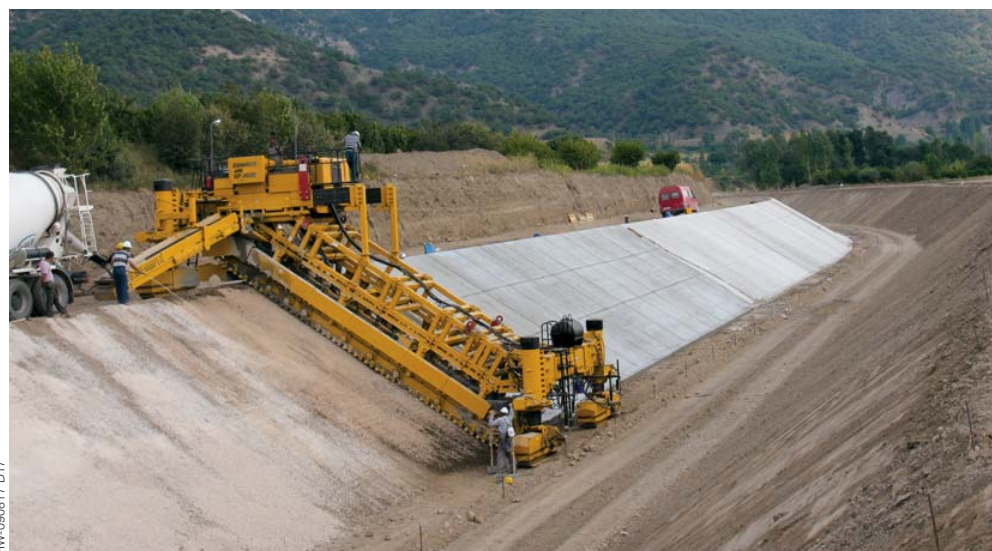
The GP-2600 paved each of the canal slopes are 9.3 meters (30.5 ft) wide.
