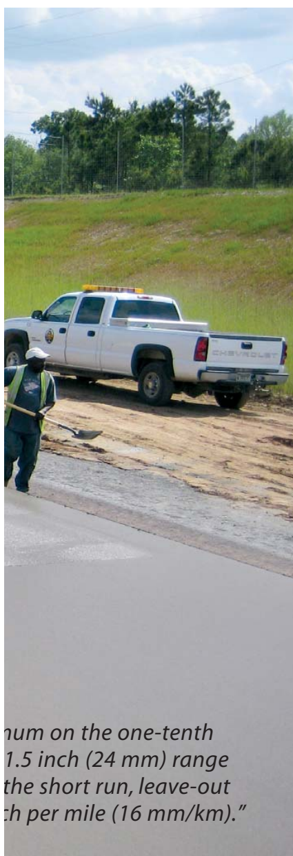
A GSI followed the paver providing instant rideability readings.
