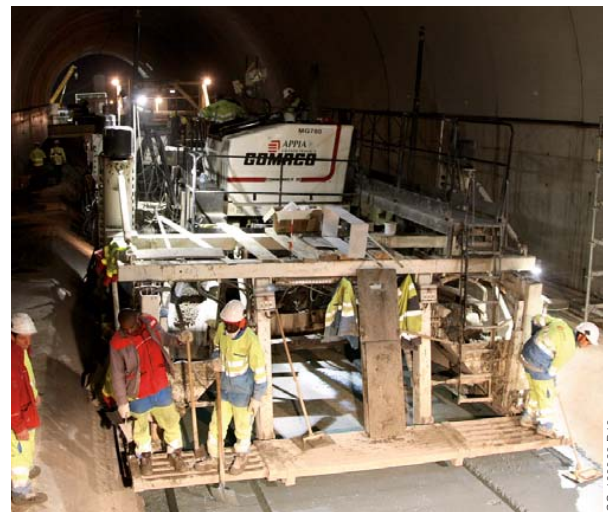
The tunnel floor was 5.6 meters (18.4 ft) wide and has an average thickness of 600 millimeters (23.6 in).
