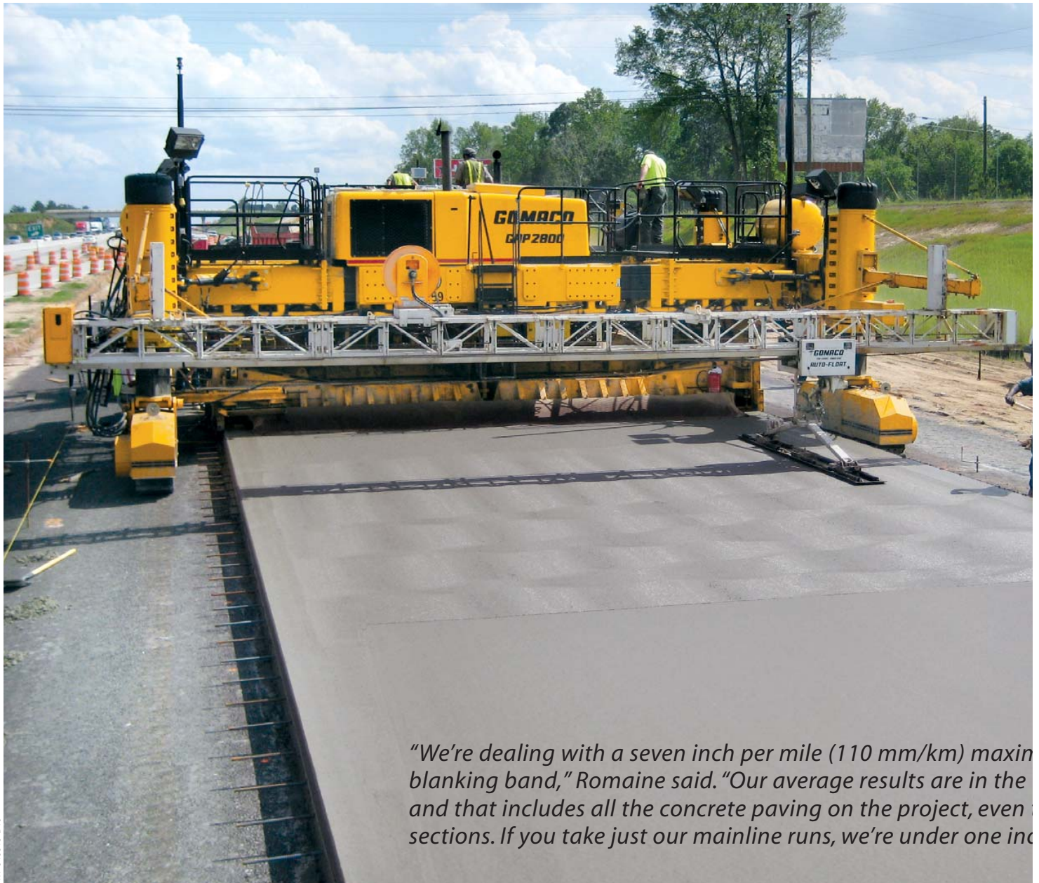
Scruggs PS-2600 placer/spreader and GHP-2800 paver are guided by the Leica stringless system. The GSI and T/C ran on stringline.
