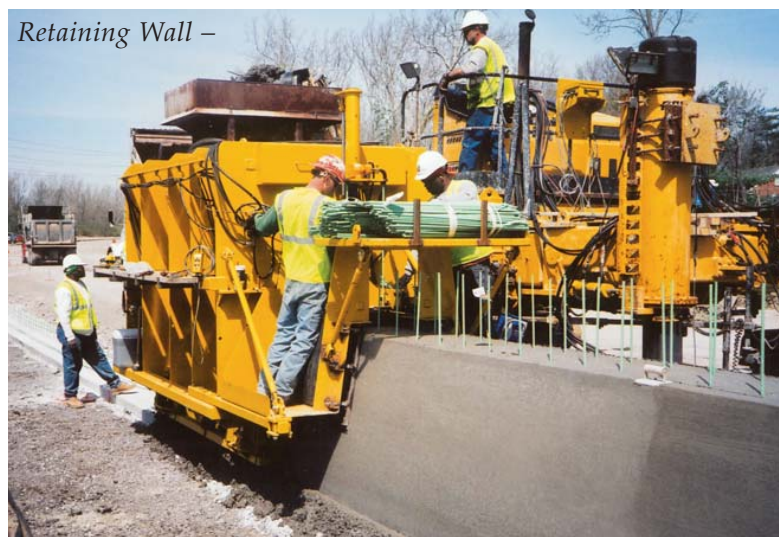
Two rebars at a time are hydraulically inserted into the top of this barrier. Another wall will be slipformed on top to form a retaining wall on the project.
