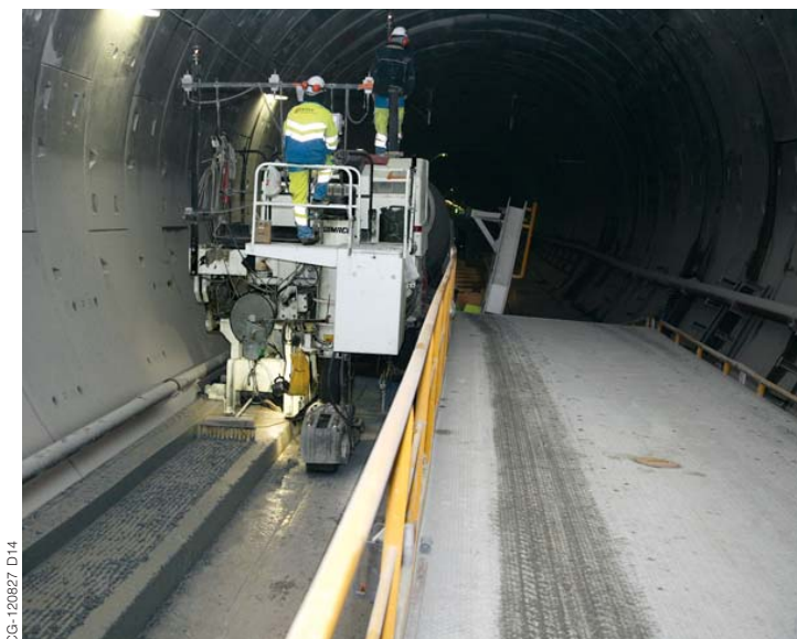
Trucks carrying concrete entered the tunnel from France, drove up and over the ramp, unloaded, and exited towards Spain.
