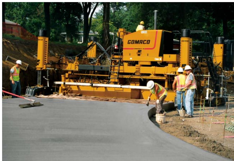
A roundabout on the project was slipformed 20 feet (6.1 m) wide with integral curb around a 45 foot (13.7 m) radius.
