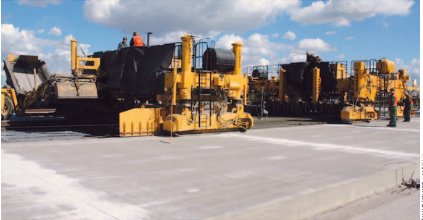
A GOMACO paving train slipforms a new 197 feet (60 m) wide runway at Pulkovo Airport near St. Petersburg, Russia.
