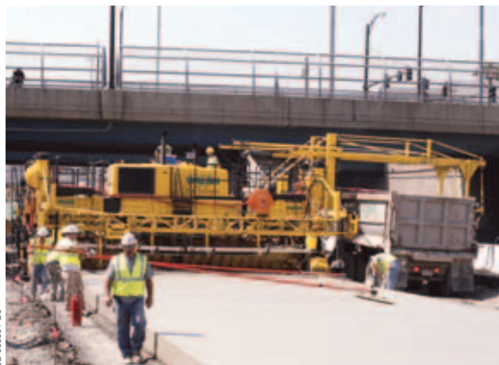
Walsh's GHP-2800 paver with hydraulic gantry system, fully extended, is running off stringline as it approaches the bridge.
