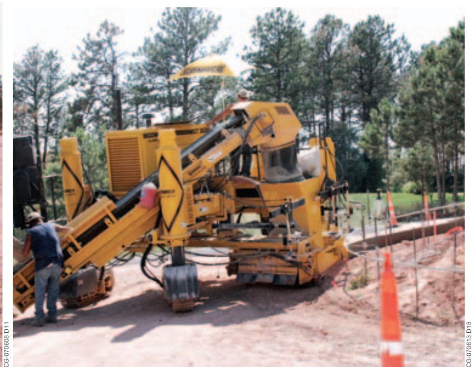
The GT-3600 maintains grade and steer while slipforming down a 14 percent slope and then transitions into a radius at the bottom of the slope.
