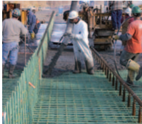
A five foot (1.5 m) wide strip for the bridge's median barrier had to be hand finished by two laborers on the project.
