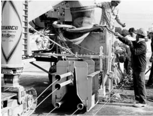
Photo #5 – Continuous reinforcing steel
