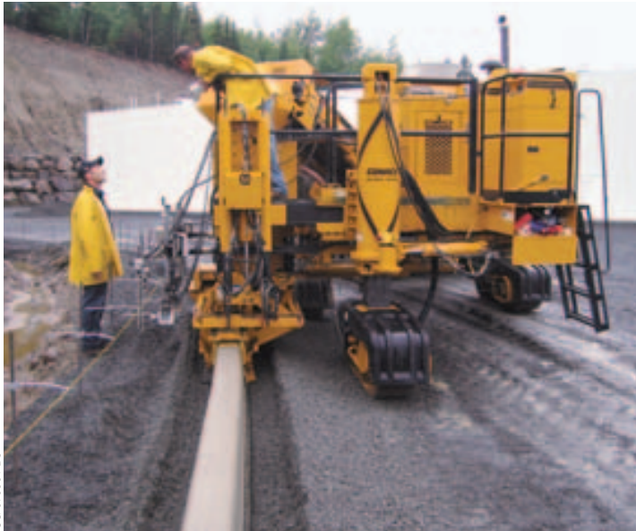
Maska Paving slipforms 16 inch (406 mm) tall ribbon curb with their GT-3600 in Montreal, Quebec, Canada.
