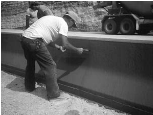
Photo #7 – Little to no handwork required
