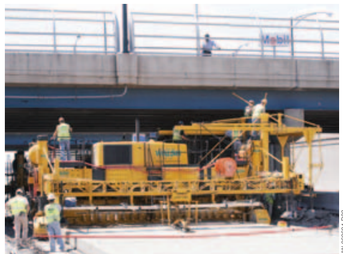
As the paver heads under the bridge, there's no clearance for the gantry system and it has to be hydraulically pulled in.
