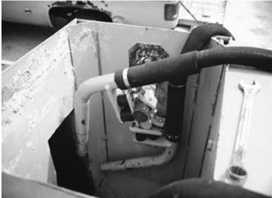
Photo #1 – Placing your vibrators
