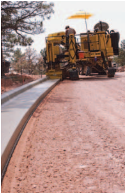
Tru-Form is slipforming a 32 inch (813 mm) wide gutter with 12 inch (305 mm) curb back.
