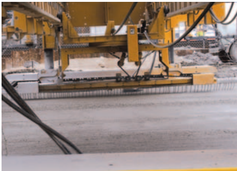
A simple sprocket and chain mechanism slides the tining rake for the skewed pattern.
