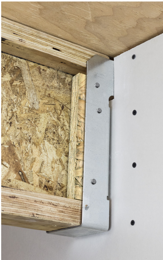
DG Hanger with I-Joists
