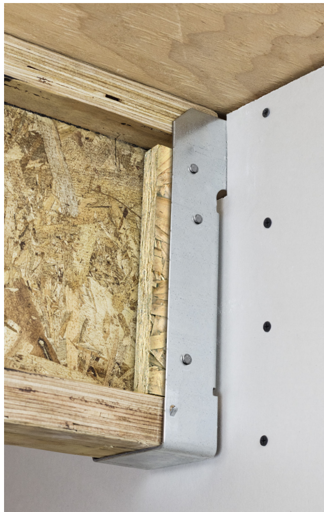
DG Hanger with I-Joists
