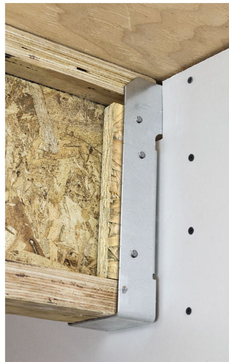
DG Hanger with I-Joists
