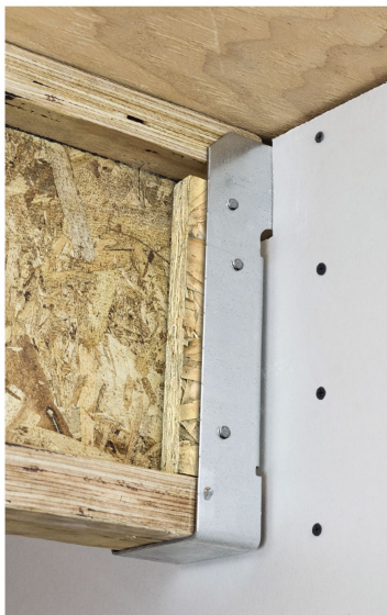
DG Hanger with I-Joists
