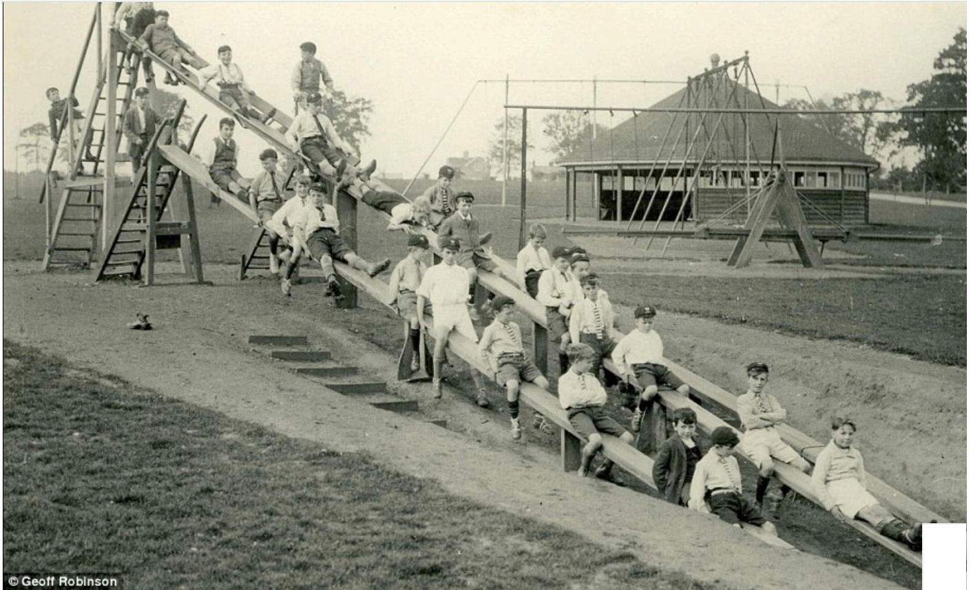
The original: The slide built in 1922 at Wicksteed Park, Kettering, Northamptonshire. Three long plans with nothing to apart from at the top of the tallest, which is 13ft high
