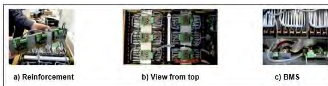
Figure B-1: Impressions of the test dismantling of battery system A
