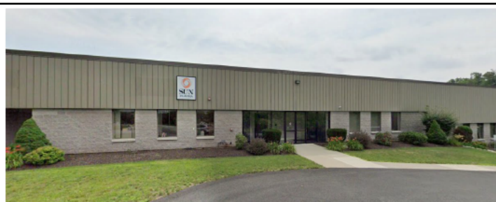
Fig. 2: Billerica, Massachusetts Facility
